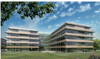
Banessa Business and Technology Park, Bucharest, Romania Design Office: Injineriile structurale Srl
