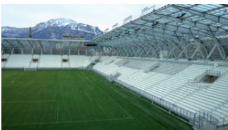
Grenoble Stadium, France Design Office: CTE SA Mulhouse Architecture Office: Chaix & Morel et associés, Paris
