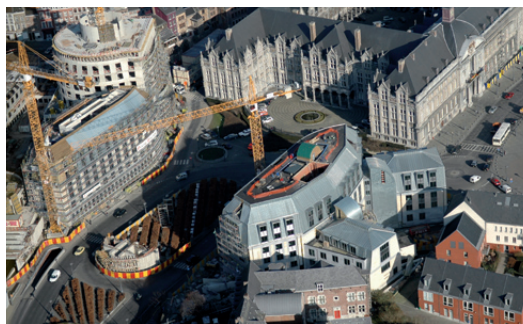
Liège Courthouse's expansion (Belgium) TPF Engineering Design Department
